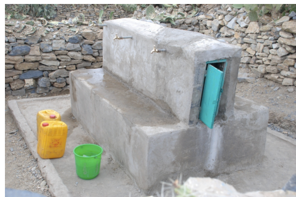
Figure 5: The new Nebar Ketema Waterpoint with adjacent jerrycans.
